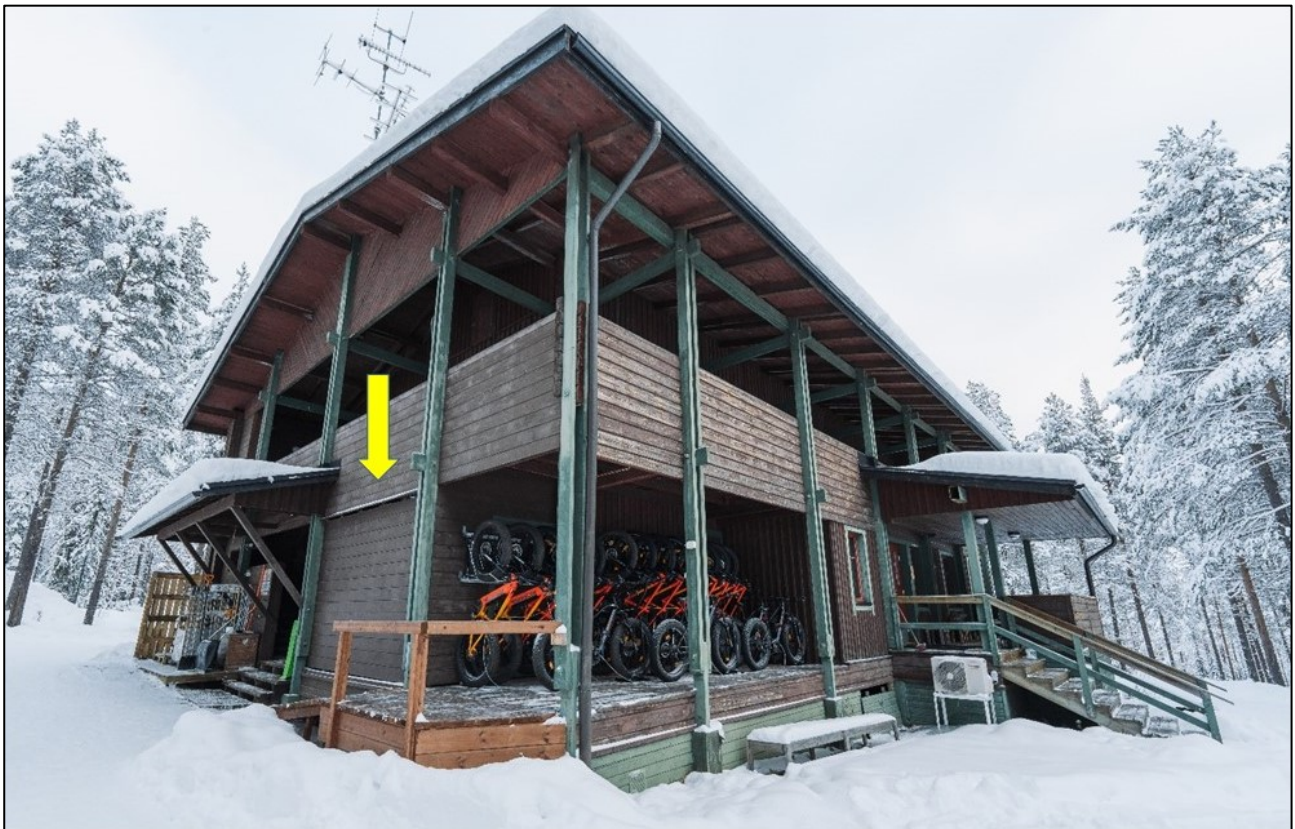
Figure 3. Hostel building from the west. The arrow points to the unheated outdoor storage area. The stairs leading to the balcony access corridor are on the left. (Photo: private person)
