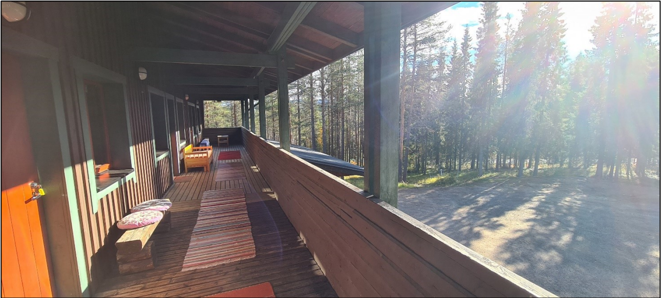
Figure 9. Doors in the first floor the corridor with balcony access looking to the southeast. (Photo: private person)
