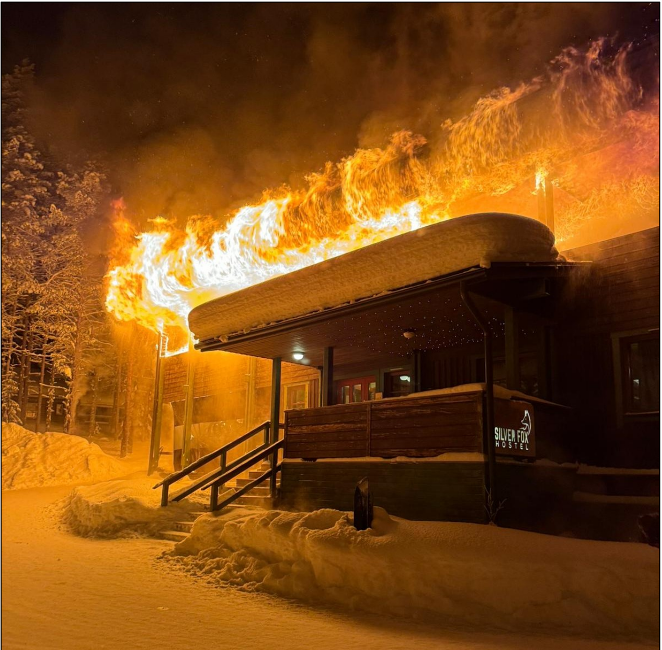
Figure 2. One of the earliest photographs of the fire. The fire spread quickly to the first floor balcony access corridor. At this stage, some of the persons who escaped were still inside the building. (Photo: private person)
