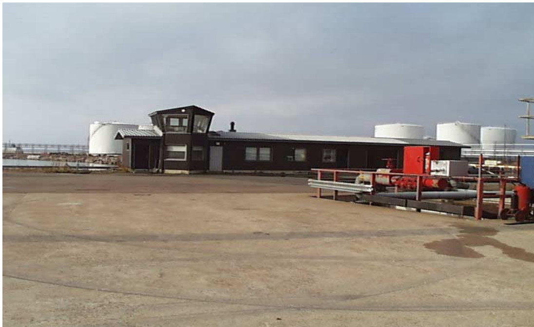
Figure 12 Control room of the representative of the terminal supervising the loading on the second floor. The room below is for the port supervisor. The pier is equipped with oil prevention gear (oil barriers and boat), not in the picture.
