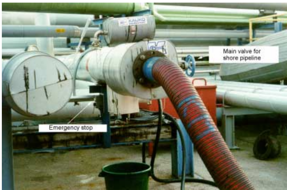
Figure 2 The loading hose, attachment on the pier, main valve and emergency stop button. Note incomplete attachment of the flange.
