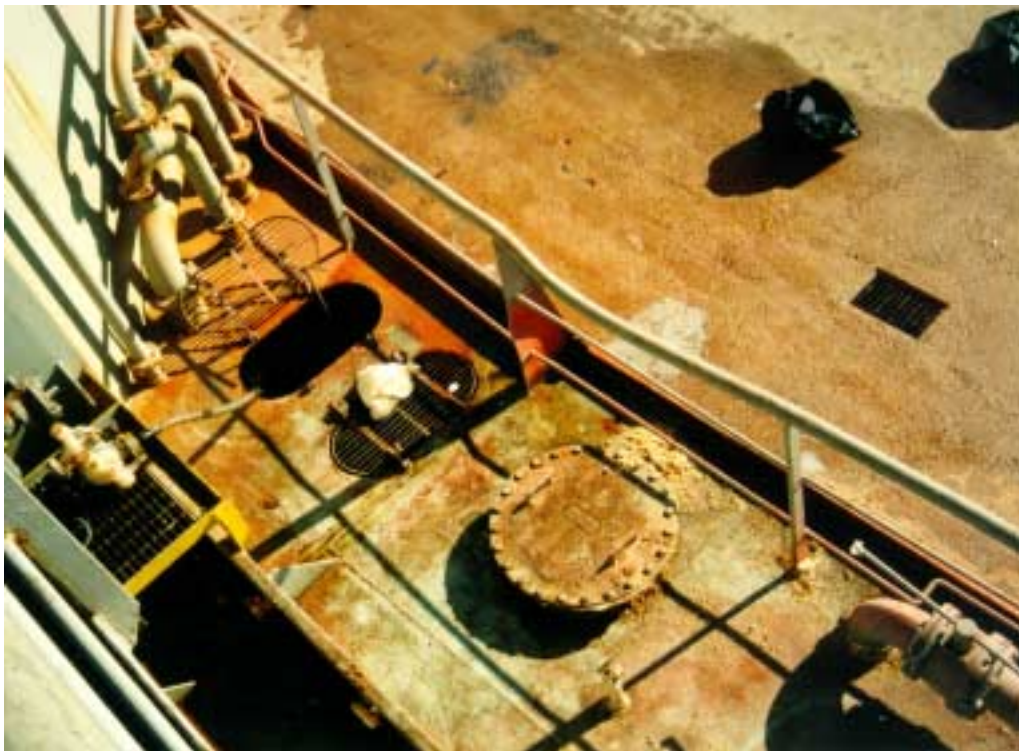
Figure 7 Ullage drain at the stern of the vessel
