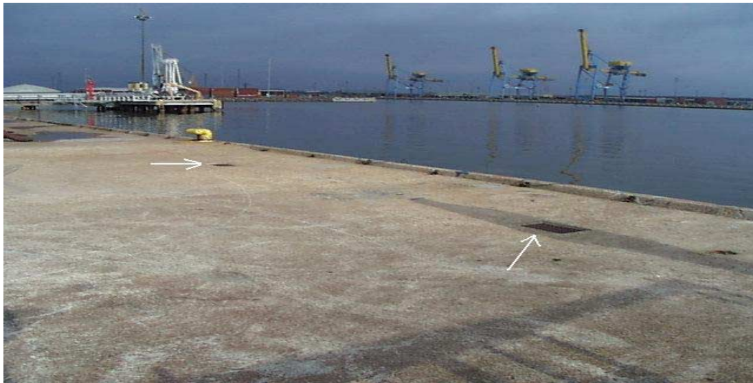
Figure 4 South end of Pier 2
