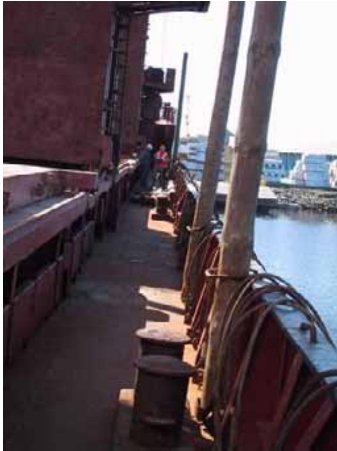
Figure 9. Installation and placement of the uprights on M/S FJORD PEARL, May 2002
