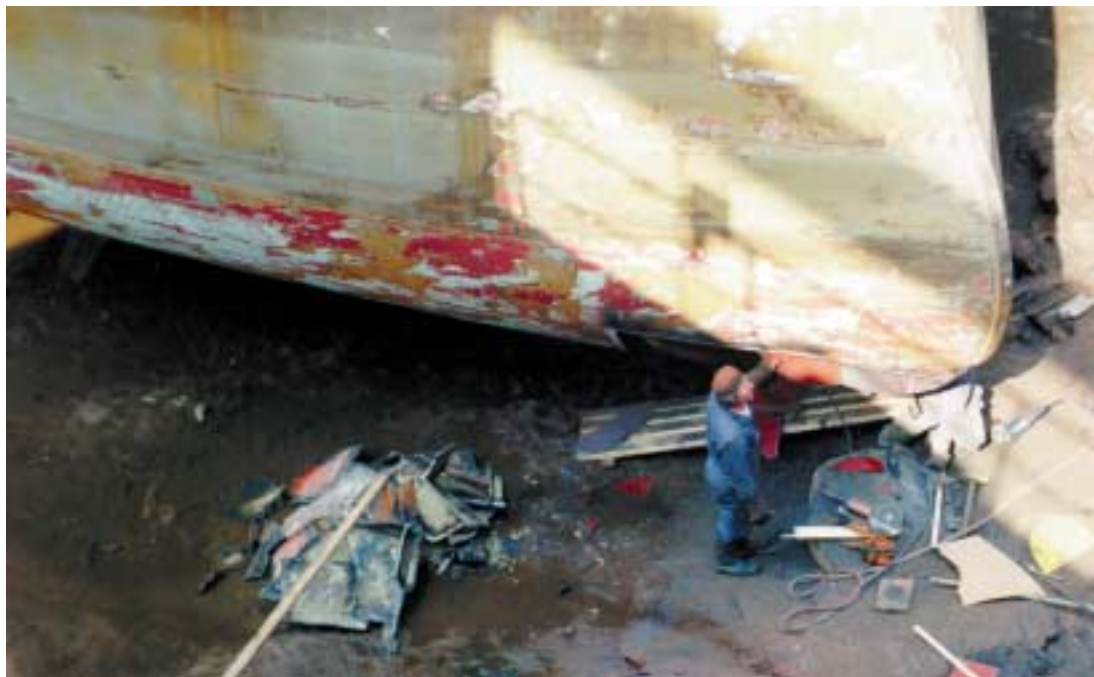
Figure 4. Damaged forepeak of ms BALTIC MERCHANT under repair at Savonlinna dock.
